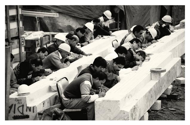
Figure 67 - Semiskilled craftsmen etching the drawings onto the marble
