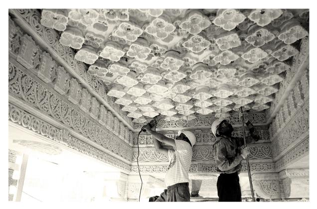
Figure 73 - Pneumatic eroding machines along with electric grinders used to do the final touches
